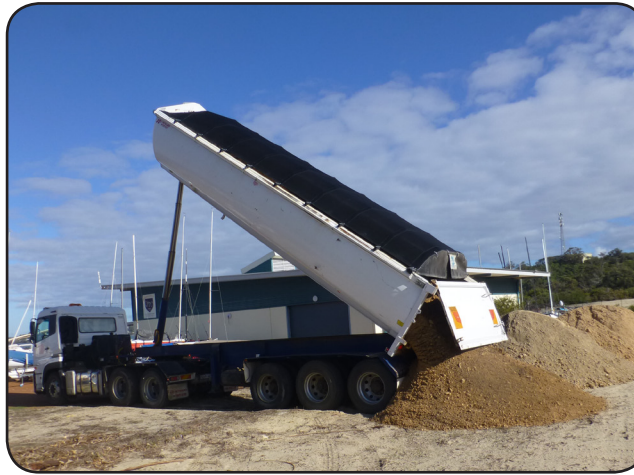
Semi trailer truck delivering the limestone roadbase. Approximately 30 loads are needed
